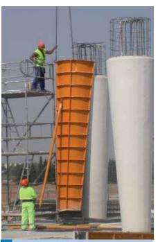
This peculiar building required unique solutions. Like the rounded forms achieved through the use of formworks made especially by ULMA Construcción for this specific work. These products were used on climbing systems to reach its 70 m. The work in heights required small intermediate forges carried out with OC shorings and BRIO Multidirectional scaffolds.
