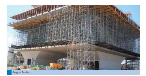
This building required high doses of innovation, since the perimeters fill was not finished. The professionalism and experience of ULMA Construcción's technicians allowed for an effective solution: to install a resistant cantilever to support the structure's weight and serve as a support to the material. For this we used 50,000 m<sup>3</sup> of OC shorings and a fast and safe assembly which was then applied on most works.
